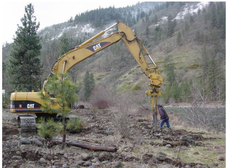
Hydraulic stinger planting the river bank on the Lower Klickitat River.
