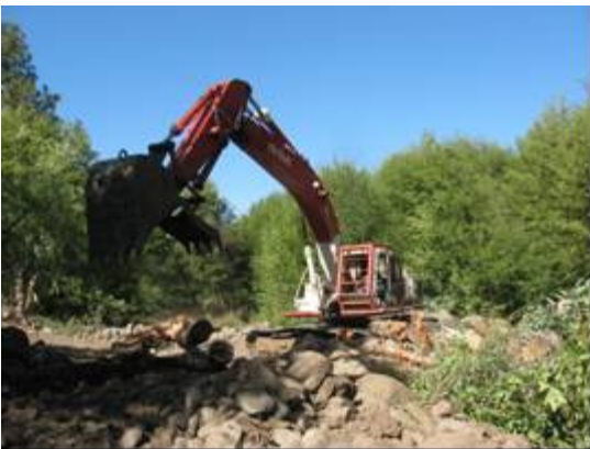
Excavator placing logs on Swale Creek, 2008.
