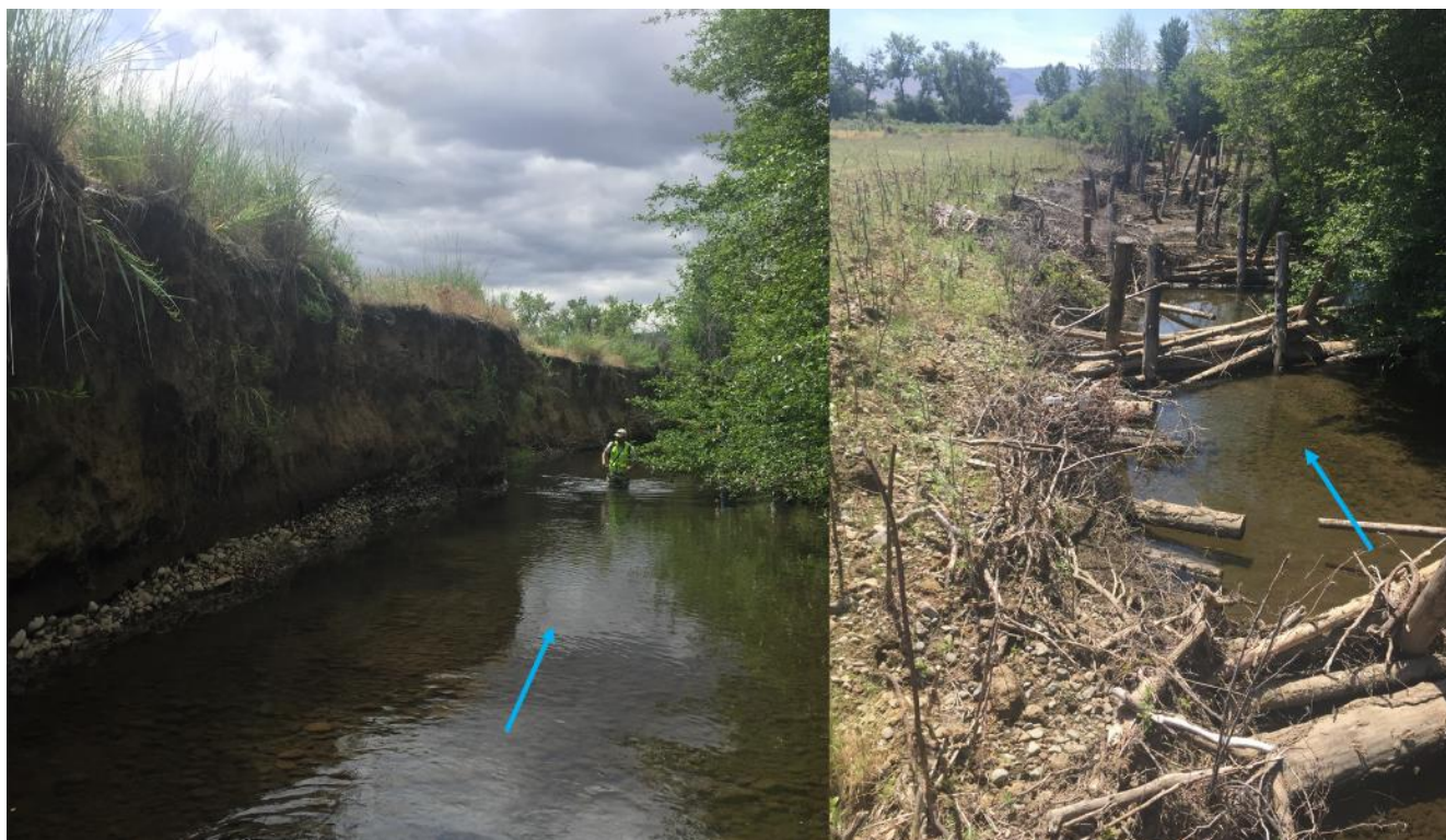
Figure 30. Example of before (L) and after (R) Valley Reset Large Wood Restoration in Toppenish Creek
