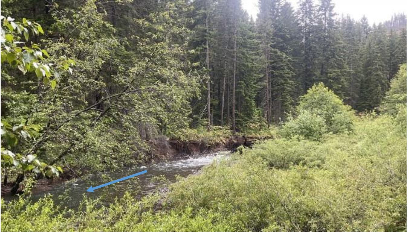
Figure 22. Example of Eroding Bank near RM 5.1 in the Middle Fork
